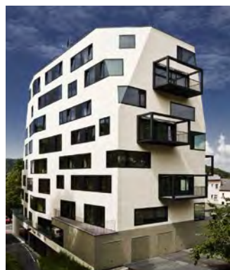
Triplex – Apartment block, Karlovy Vary, Czech Republic
