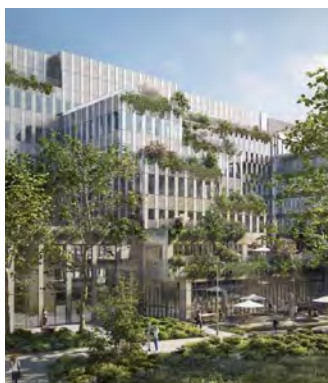
UBS Pleyad Business Centre Saint-Denis, France
